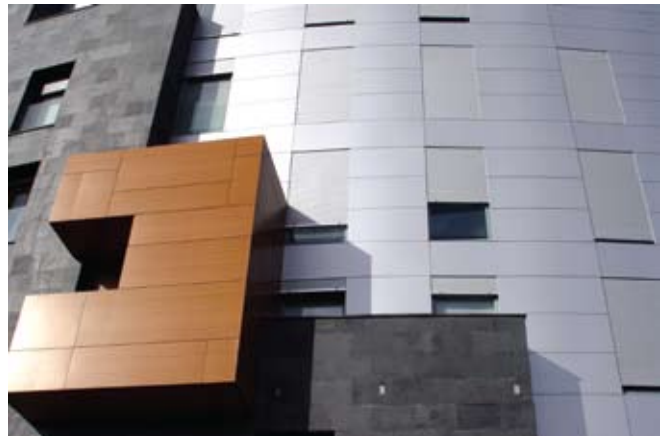
Residence Building Piedras Blancas (Spain)
